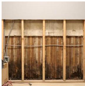
*Water damage to the walls of the Sumas police station give stark evidence of the deep and lingering flooding the town experienced late last year when the Nooksack River breached its banks. Much of the community is still working to rebuild and recover.*
